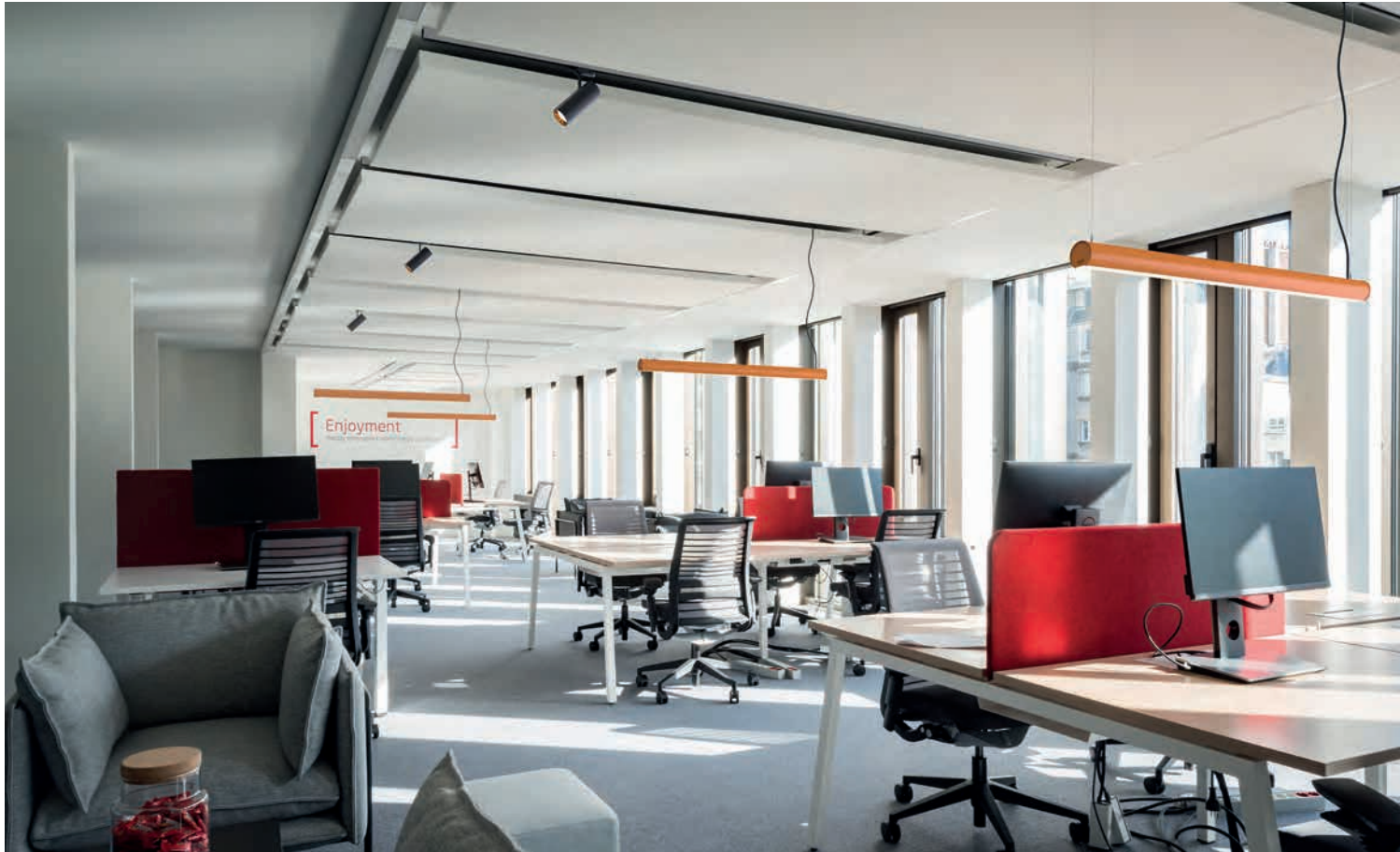
Spaces with semi-concealed installations (large format acoustic panels).
